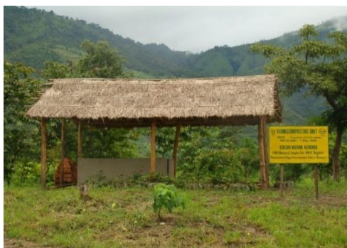
Thetch roof shed
