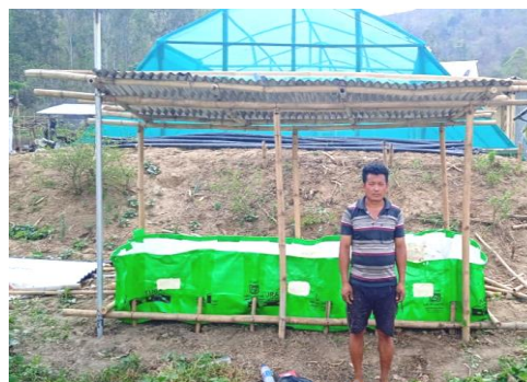
G.I Sheet roof shed
